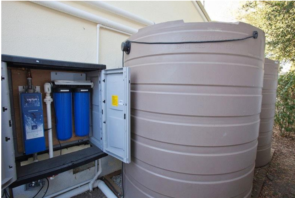
An 865-gallon rain barrel next to a water filter and micron filters for harvested rainwater on a green home in Los Angeles. (Citizen of the Planet/Education Images/UIG via Getty Images)
